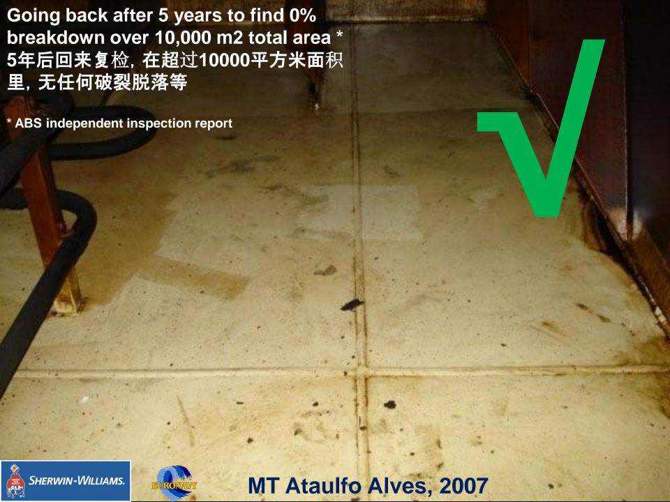
Do it with hydroblasting, without dehumidifier and over flash rust (WJ2M). Again...
