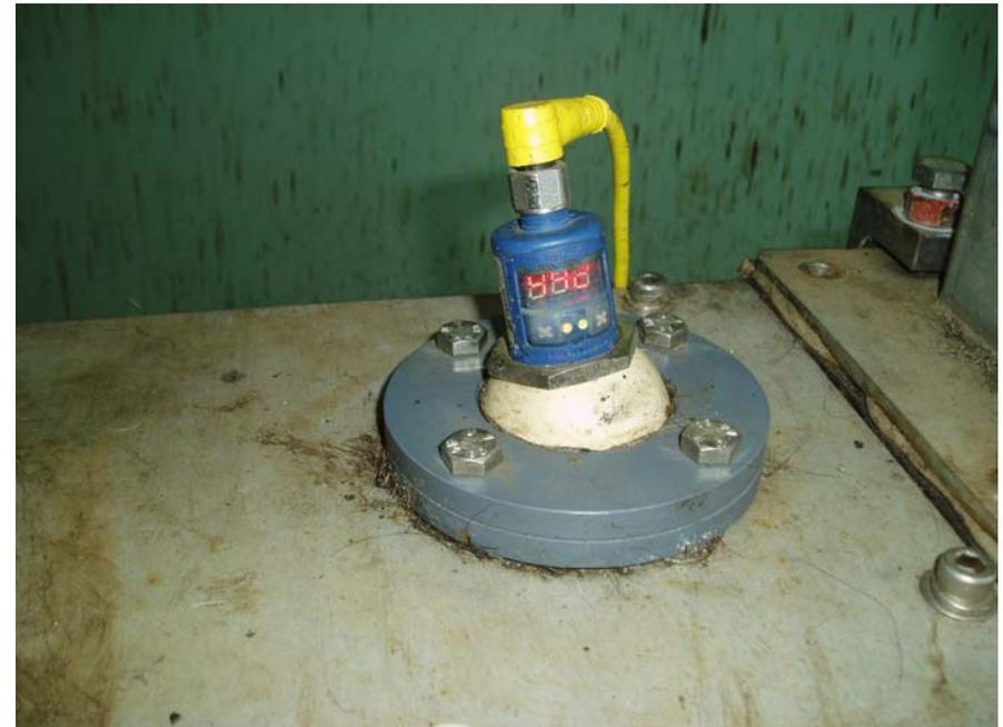
Sludge level control with an ultra sonic sensor
